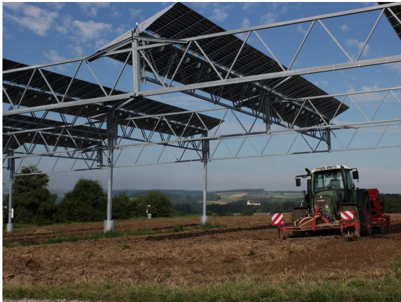
Figure 2: Agro-photovoltaic system of the Hofgemeinschaft Heggelbach 13 . Agricultural production and energy production in the same place are not mutually exclusive.
